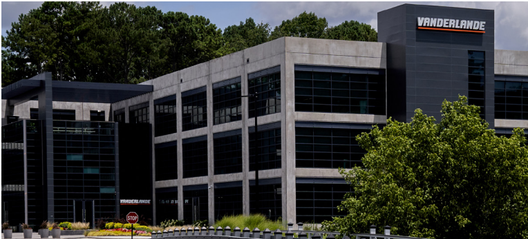
Town Center's newest office development is The Edison Chastain, home to Vanderlande Industries. It was completed in 2020 and has 152K SF of Class A office space.
