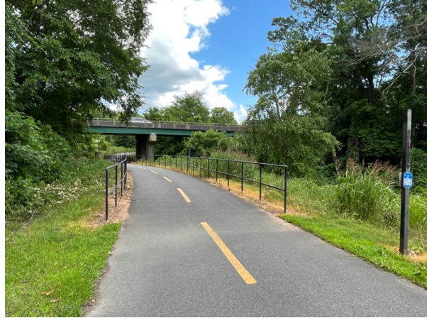
On trail looking west at approach to bridge.
