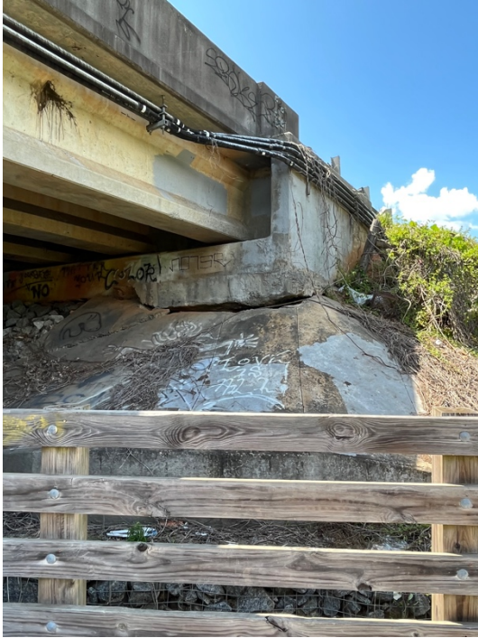
Looking northwest at bridge C and embankment.
