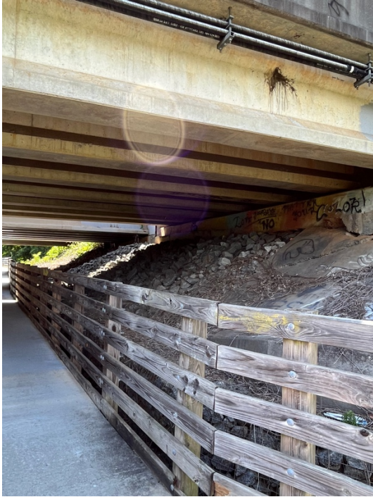
Looking west at bridge C and embankment.
