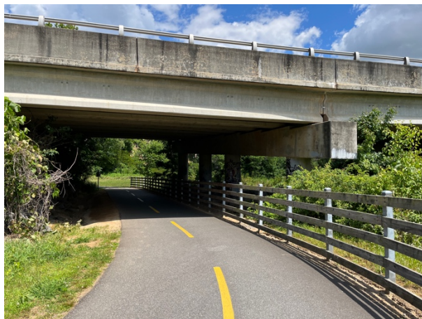
Looking east at bridge approach.
