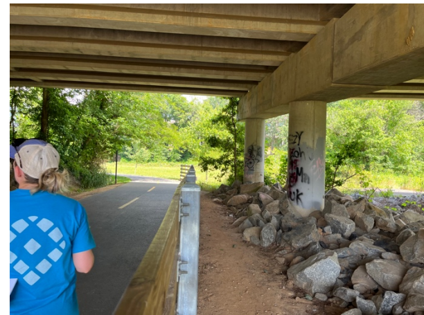
Area at back of railing.
