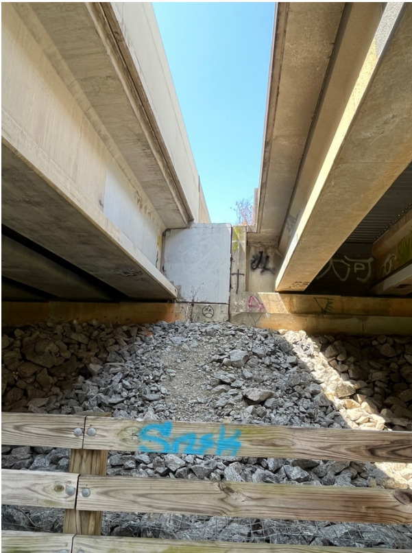
Bridge B on the left. Bridge C on the right.
