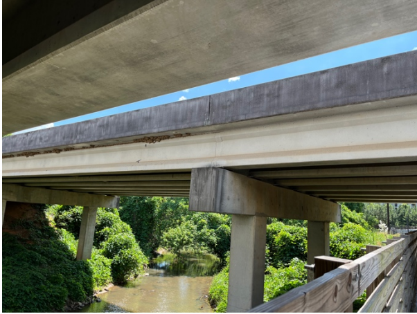
Looking back west at bridge A .
