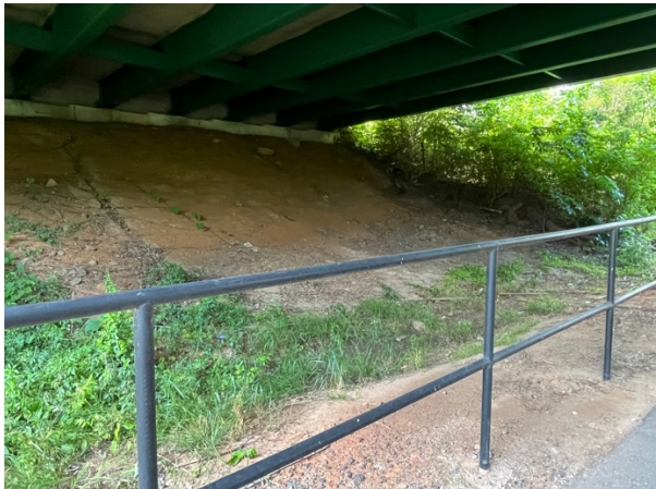
Looking north east at bridge embankment.
