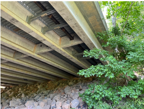
Embankment and concrete beams.
