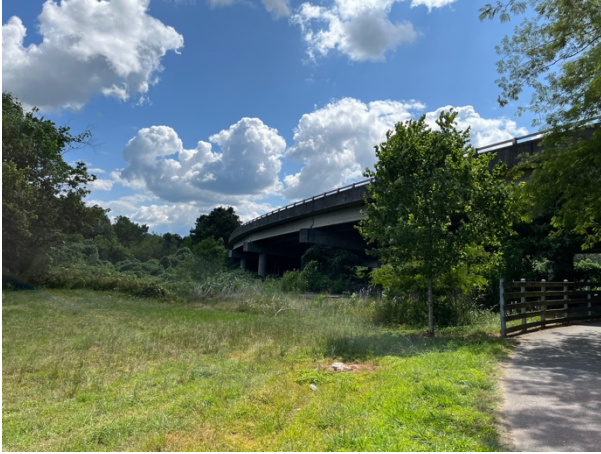
Looking south west towards bridge.
