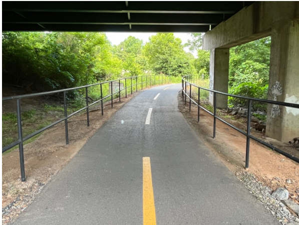
On trail looking east under I-75 bridge.
