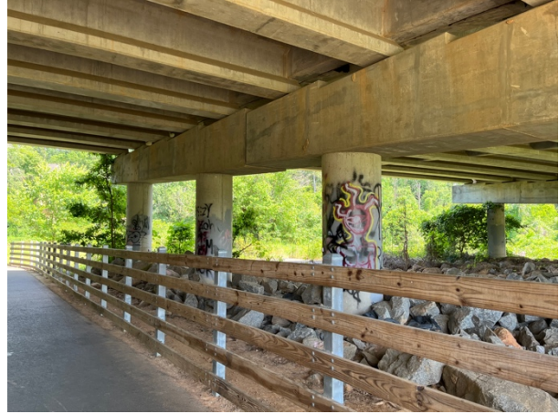
Concrete columns, supports and overhead beams.
