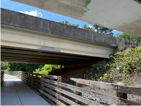
Looking back west at bridge A .
