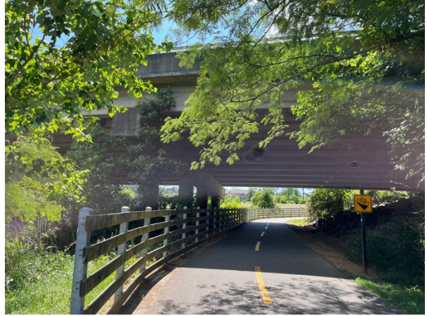
Looking west towards bridge.
