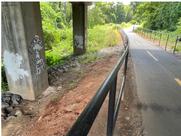
Slope from trail to base of columns.
