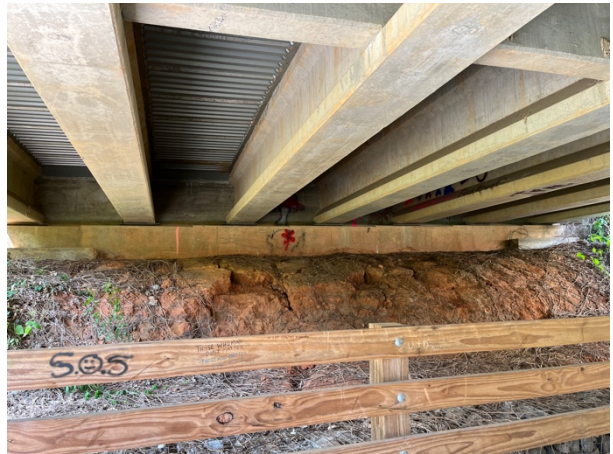
Looking north at bridge embankment. (Bridge A.)
