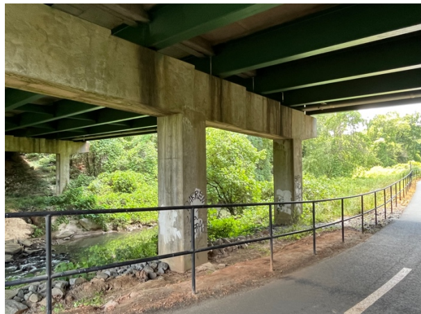
Looking southwest under I-75 bridge.
