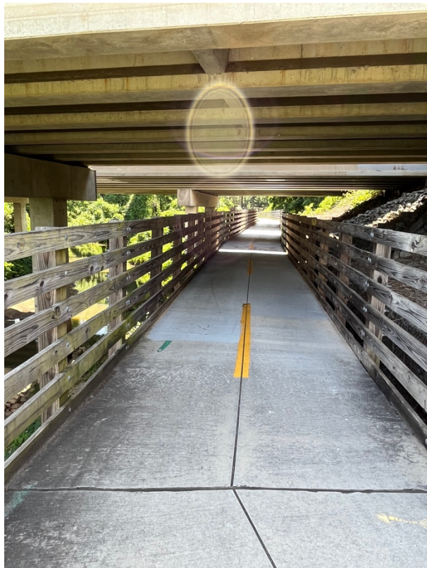
Standing at bridge C looking west under all overpasses.
