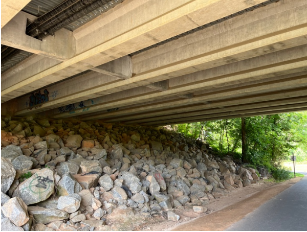
Bridge embankment and rock.
