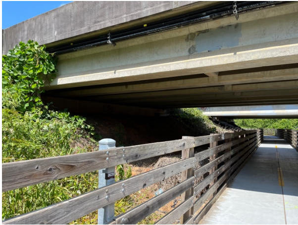
Looking east at I-575 bridge. (Bridge A.)
