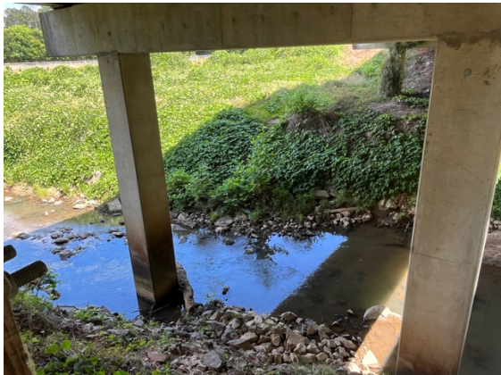
Slope from trail down to column base of Bridge C .
